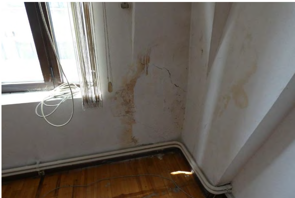
Foto 33 – Fracturi inclinate in pereti
